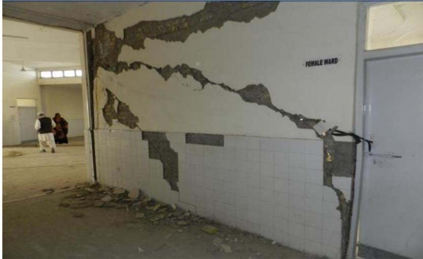
*Cracked walls in a hospital in Quetta due to land subsidence*
