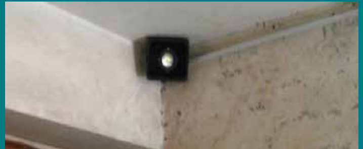
LEDs sufficiently apart from stocks
