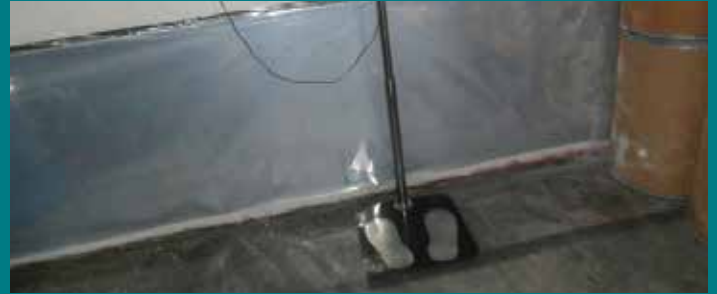
Discharge Station at ink mixing department
