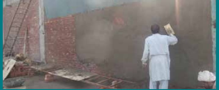
Partition wall between dispatch store and flammable chemical yard
