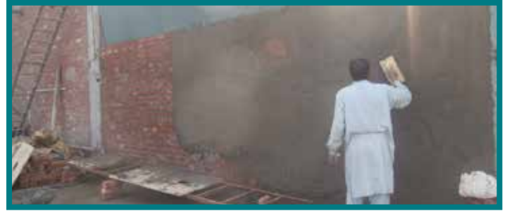
A wall partition built between the dispatch area and the flammable chemicals storage
