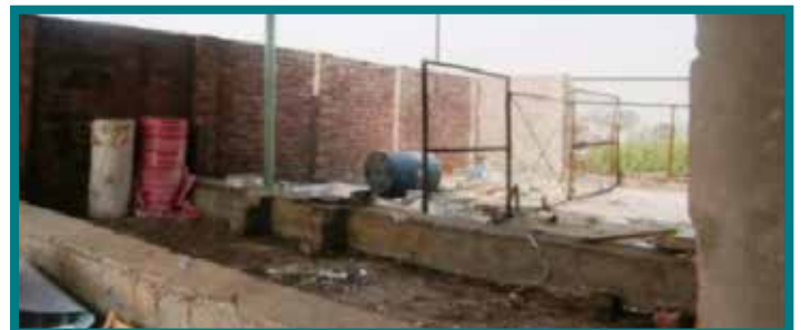
Regular waste removal at waste yard
