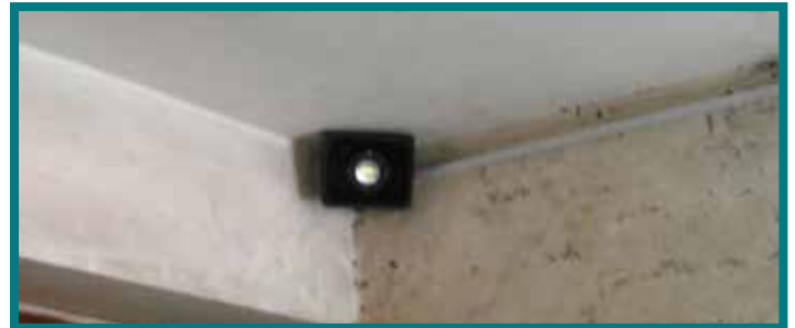
LEDs sufficiently apart from stocks
