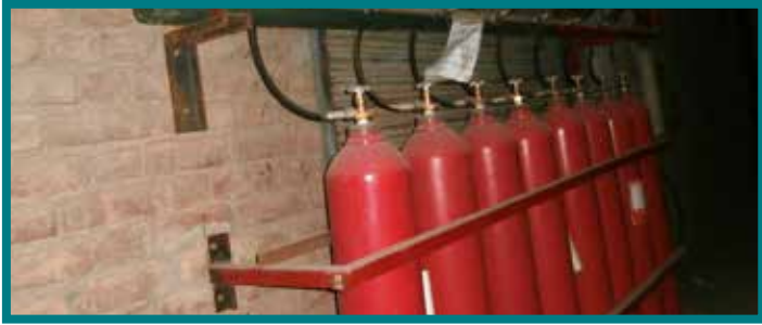
CO2 Cylinders for the suppression system
